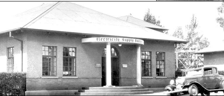
*The administrative offices of Electricity Supply Commission (Escom) at the corner of Hofmeyer Street and Smuts Avenue.
